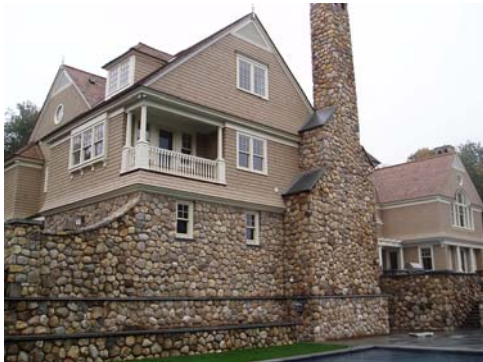
View of stone veneer and high chimney
