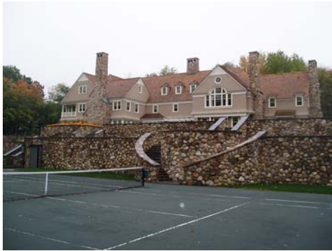
Various levels of site retaining walls
