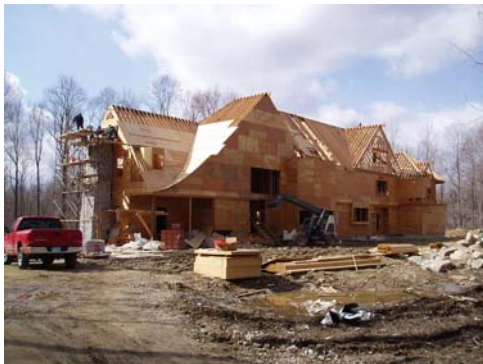
View of building under construction
