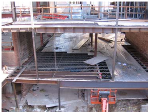
Steel framing required consideration of existing site conditions
